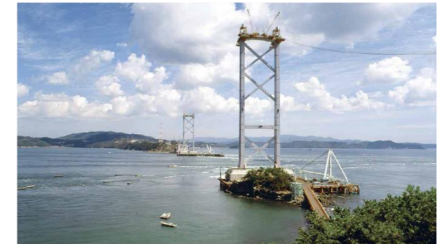
Main tower of Onaruto Bridge under construction (completed in 1981)
