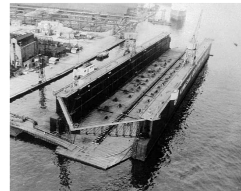
Third floating dock completed in 1953
