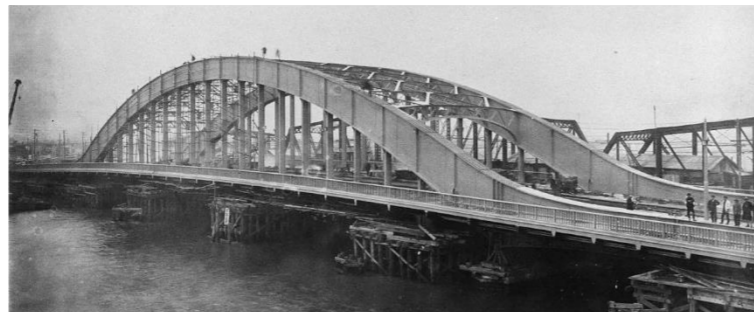
Eitai Bridge just before it was completed in 1926.
