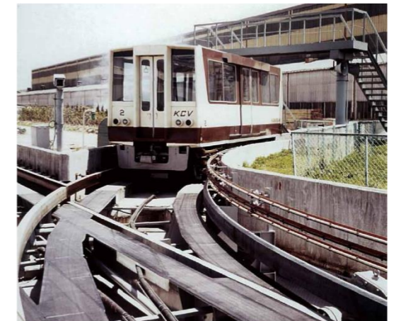
Kawasaki Computer-controlled Vehicle (KCV) system test line installed in 1974
