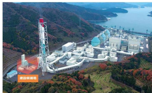
Artist's rendering of the pilot scale test facility at the Maizuru Power Plant (Photo: Kansai Electric Power Company Inc.)
