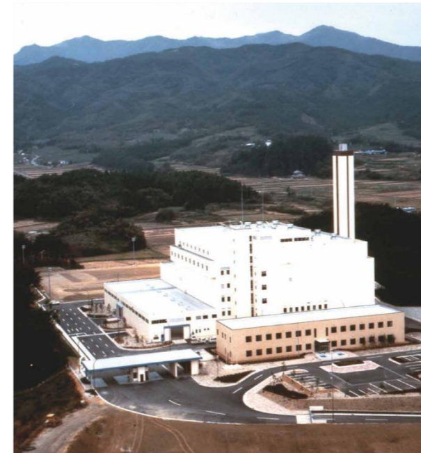
Kouzu Cleaning Center in Koriyama City, Fukushima Prefecture completed in 1984
