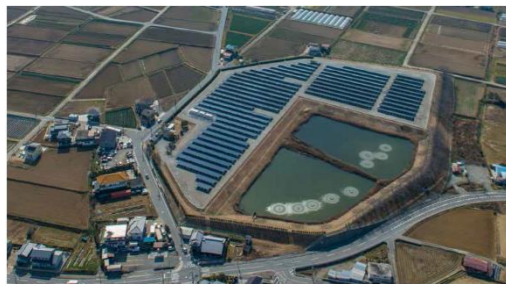
Solar power plant at the former landfill site
