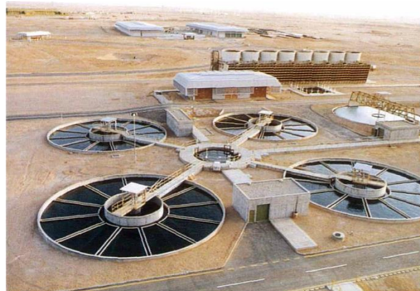
Wasia water treatment plant (Saudi Arabia) completed in 1982
