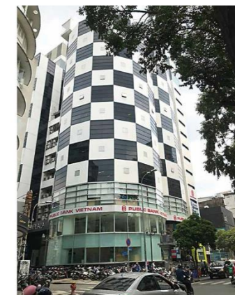
Kawasaki Motors Vietnam Co., Ltd. (KMV) office building
