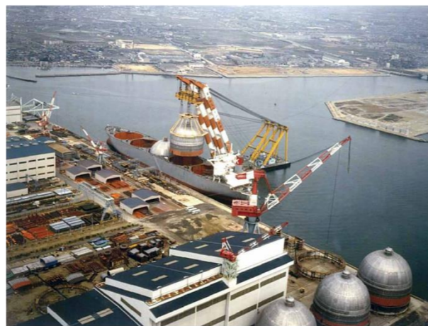
Installing tanks on the Bishumaru LNG carrier (delivered in 1983) at the Harima Works
