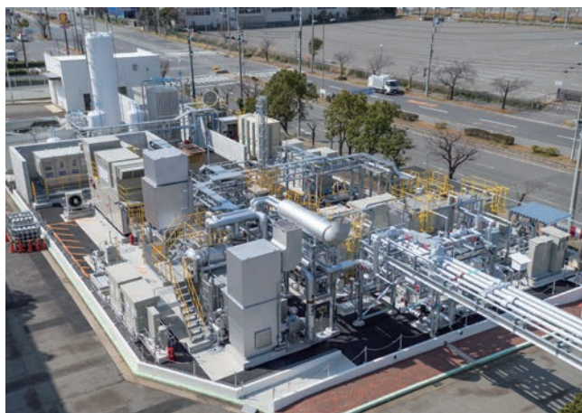
(a) Exterior of facility
