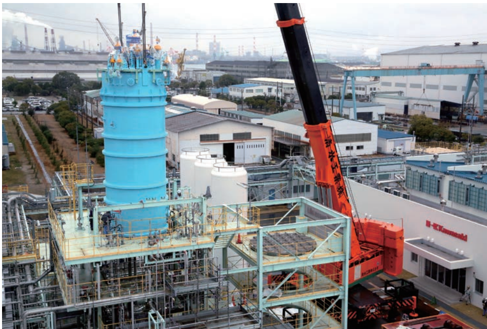
Fig. 5 Installation of new liquefier
