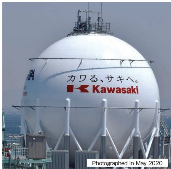
Fig. 3 Liquefied hydrogen storage tank
