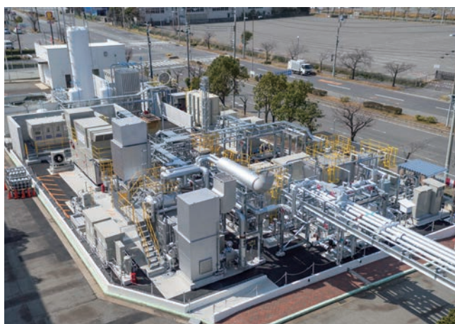
(a) Exterior of facility
